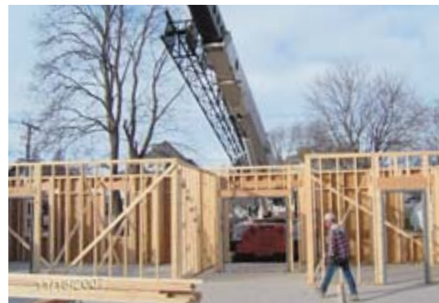
Framing the building
